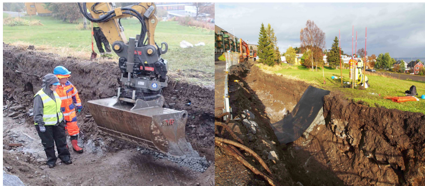
Fig. 5. (left) Securing a section with clay, lifted into the trench by the digger. It was then padded on by hand to protect the installed monitoring equipment (photograph courtesy of Michel Vorenhout, MVH Consult). Fig. 6. (right) Securing a section with clay. For the rest of the trench, the digger pushed the clay towards the section to protect the deposits from oxygen influx and dewatering (photograph by VVM/NIKU).
